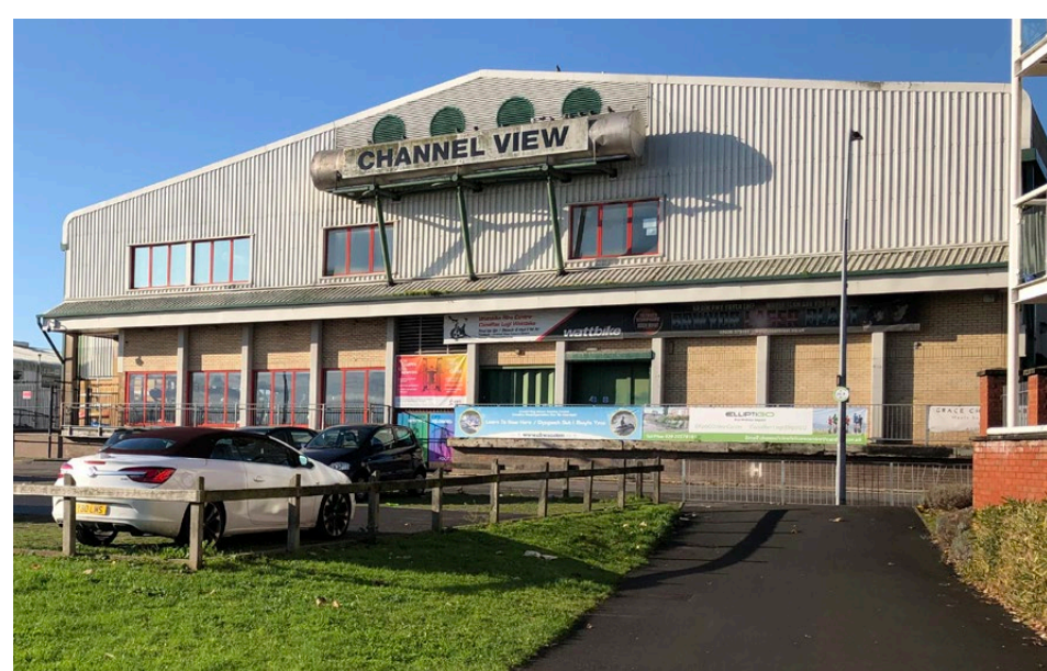
Channel View Leisure Centre | Canolfan Hamdden
